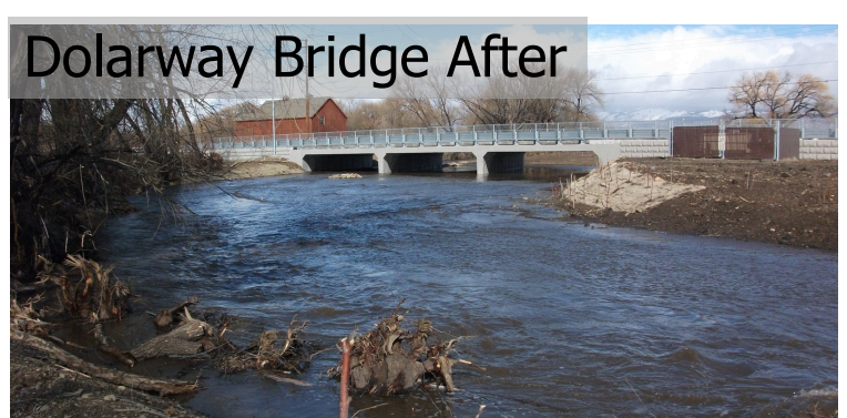
Completed Dolarway Rd. / Reecer Creek Bridge, (after)
