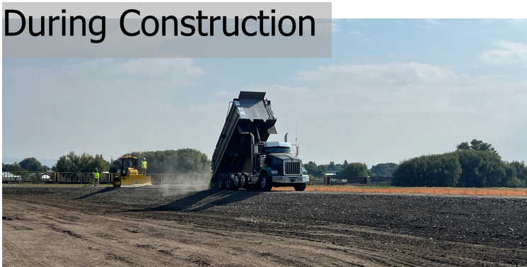
Placing gravel, Reecer Creek Levee Project, 2025
