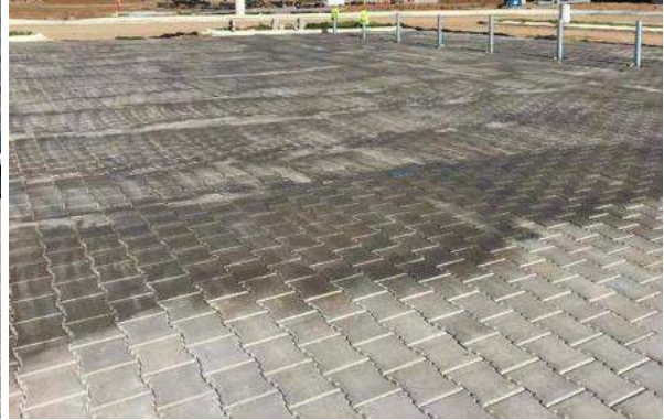
Close up immediately following sealant
