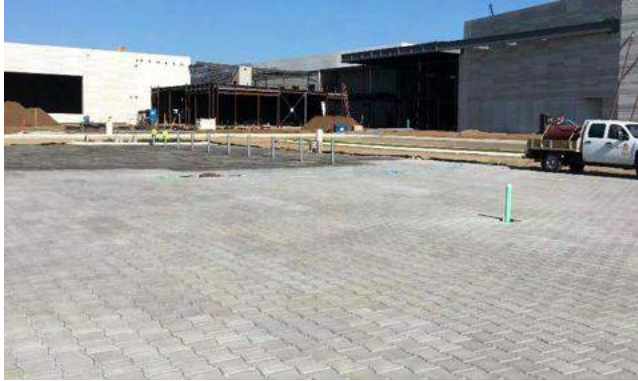
Sealant being applied on PaveDrain via Sprayer
